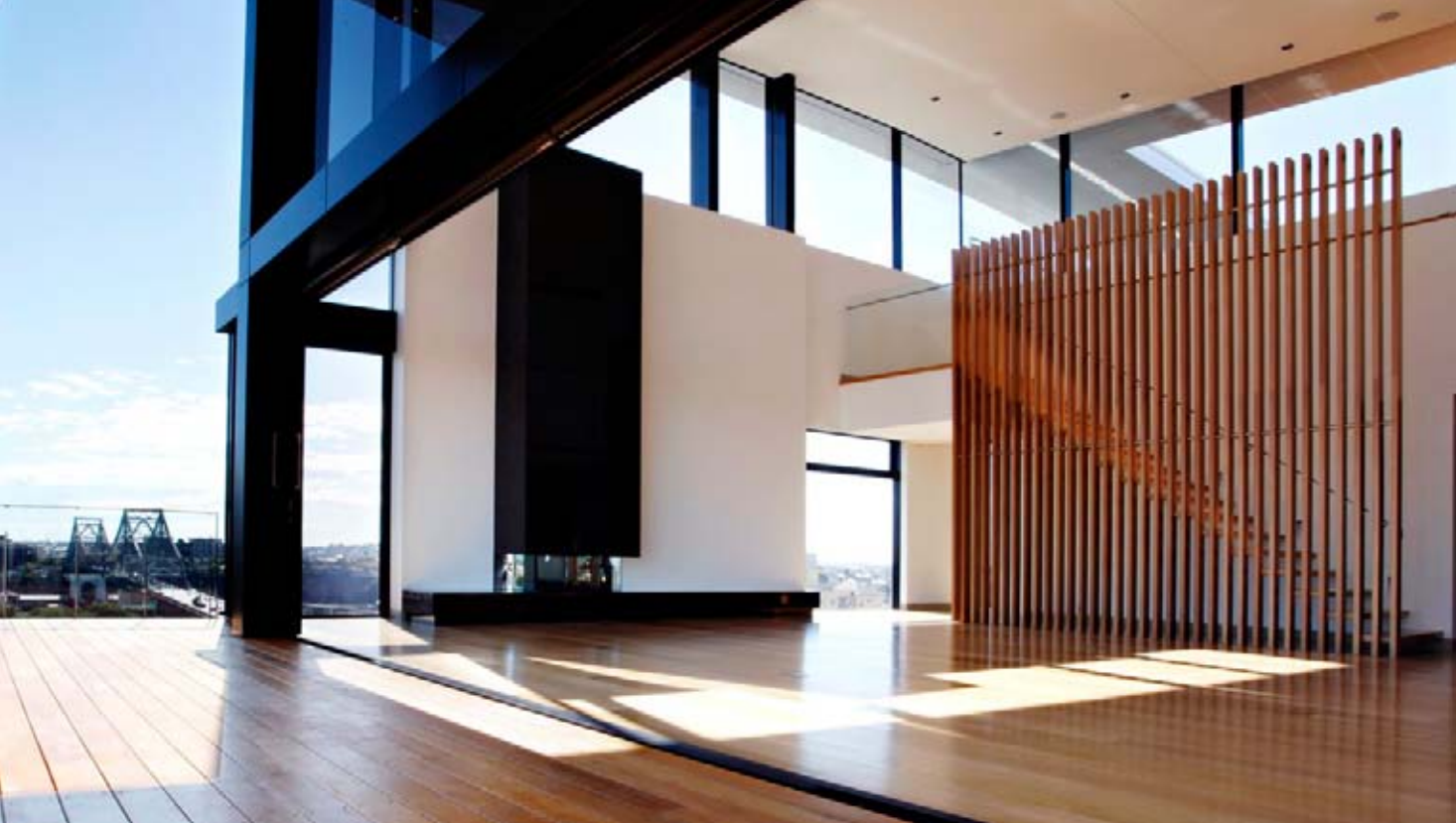
Vertical timber batten balustrade
