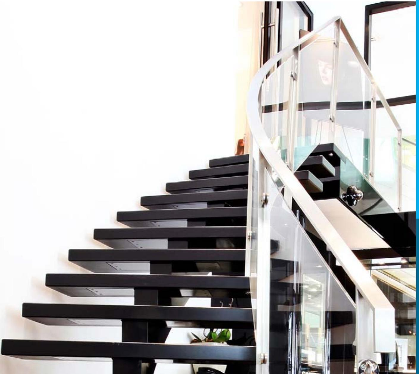
Figure 6. H4 corner balustrade section with flat-bar top-mounted handrail matching stanchion blades.
