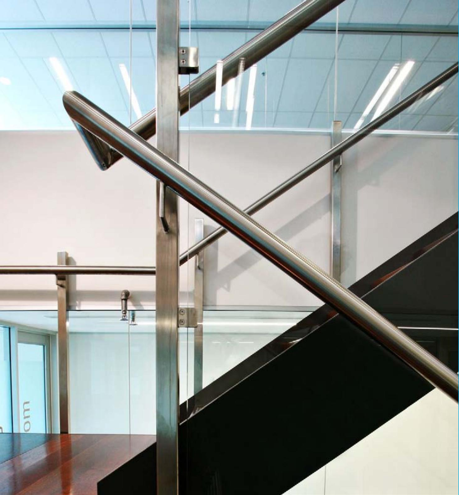
Stainless SHS stanchions with glass infill and offset handrail
