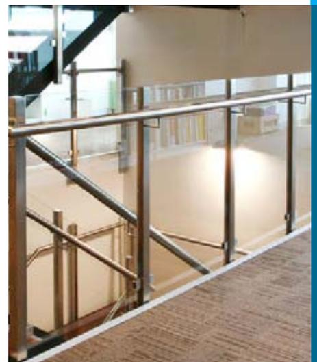
Figure 6. An alternative concealed-baseplate floor fixing method, which is preferred in most modern office designs. A concealed baseplate is also more appropriate when higher design loads are specified.
